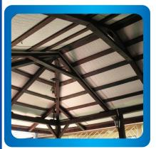
It is recommended a distance of 1.20 meters to 2.20 meters between supports.
